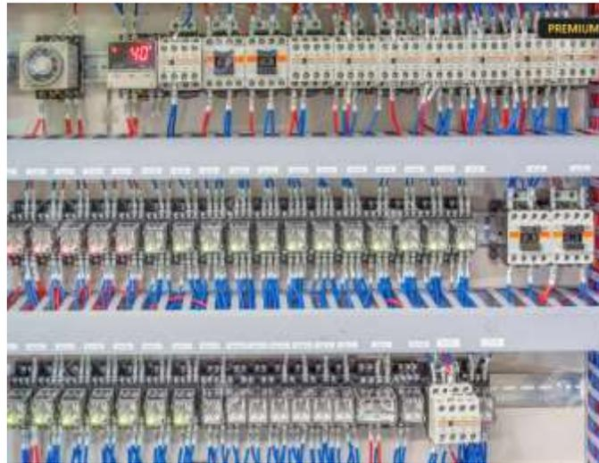
FIGURA 14: CONTROLADOR LÓGICO PROGRAMABLE (LÓGICA CABLEADA).
